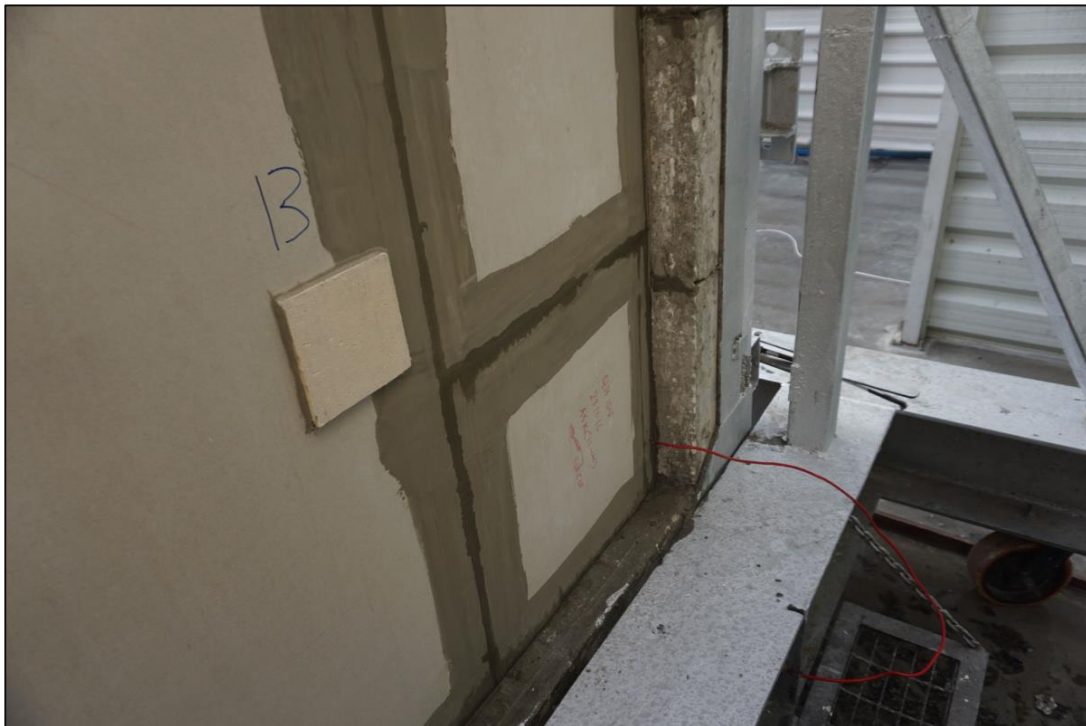
Picture 14: The extend of moisture collection on the unexposed face of the specimen immediately following the hose stream test.
