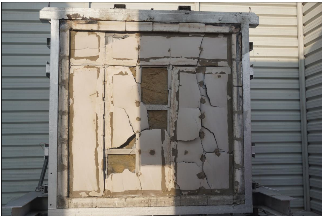
Picture 12: The exposed face of the specimen immediately before the hose stream test. =
