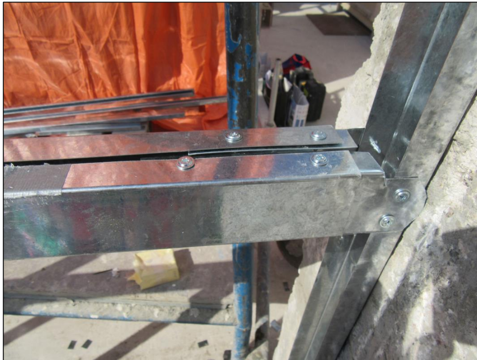
Picture 2: A photo of the tracks being used as horizontal studs and as the vertical termination stud, as well as being lengthened to fit the 3048mm wide test frame.
