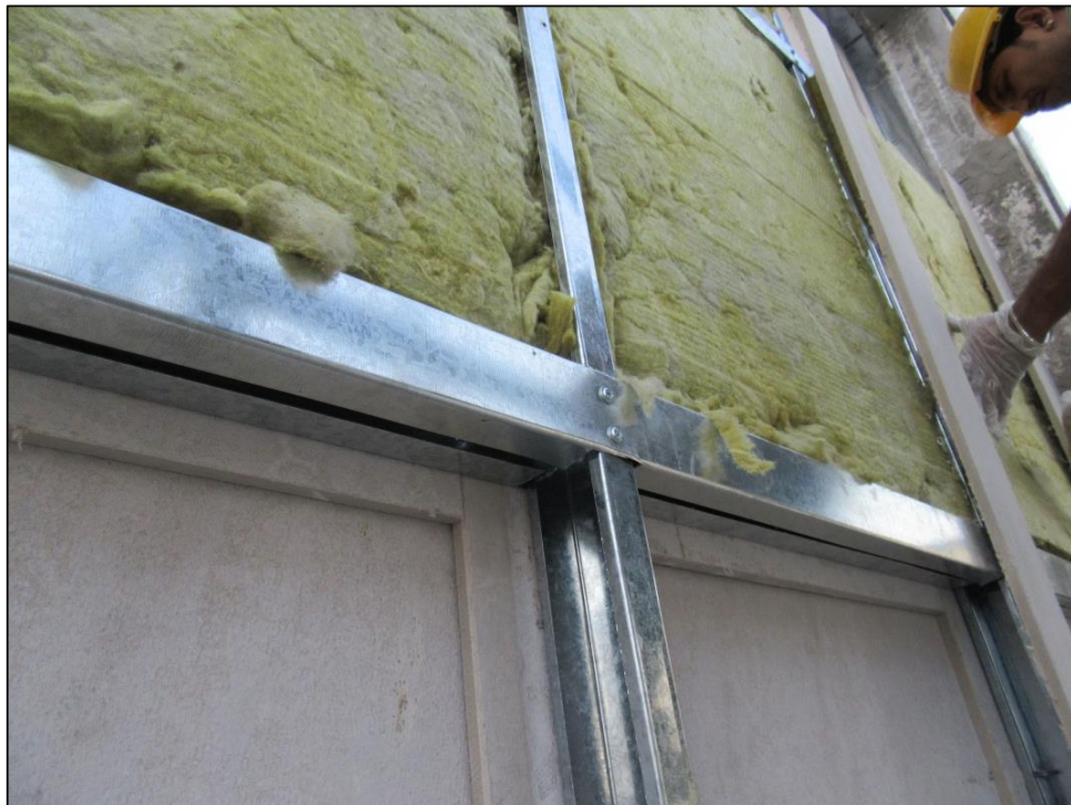
Picture 4: A photo of the rockwool insulation partially installed, as well as the 100mm wide cement board strips on both the exposed and unexposed face of the specimen.
