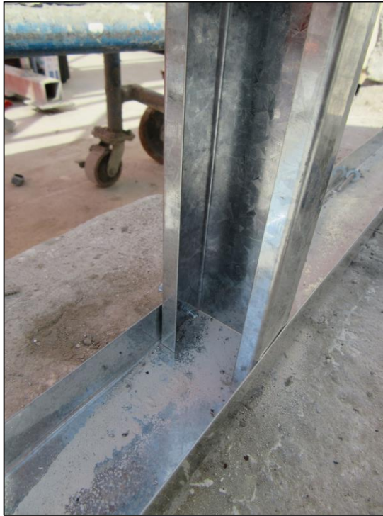
Picture 1: A photo of a vertical c-channel stud being set in the horizontal sill track.
